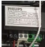
SPD to protect driver & LED Module
